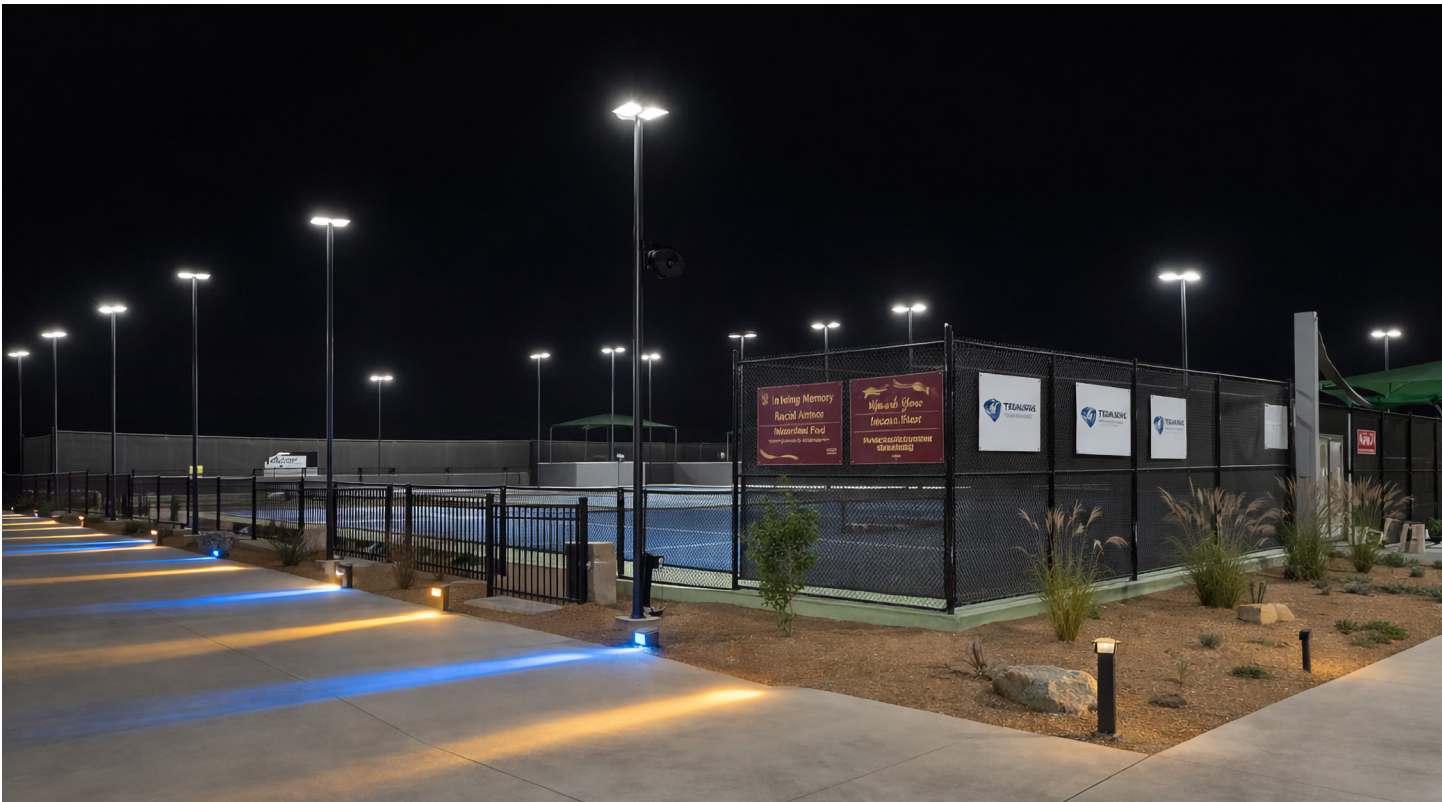
Forked Lightning Racquet Club | Santa Fe, NM Installed Lighting System: ProCourt
